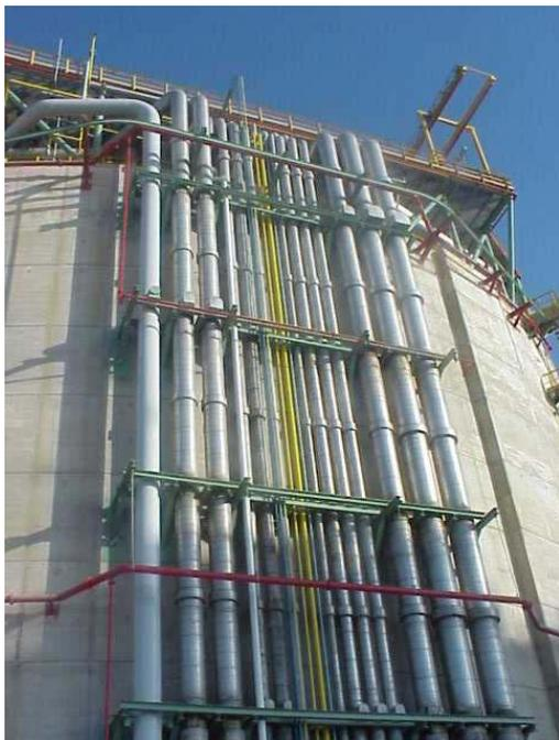
Fig. 2.14 – Tubagens do Tanque de GNL (105.000m<sup>3</sup>)
