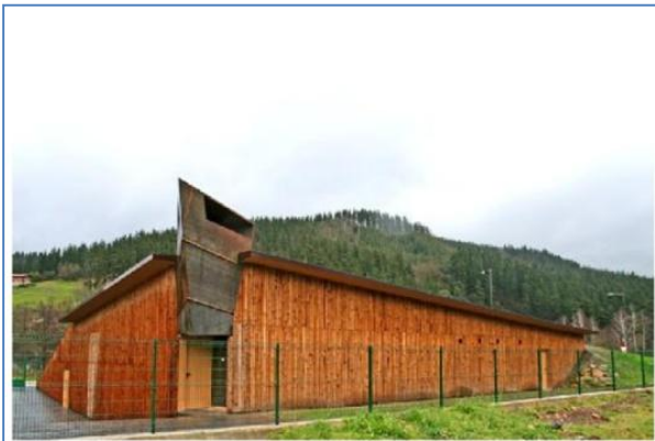
District Heating with biomass in Orozko, Spain
