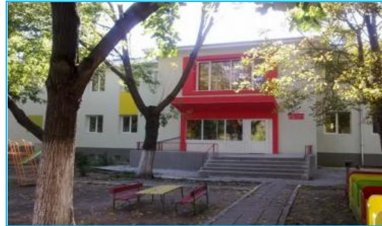
Energy renovation of school buildings in Silistra
